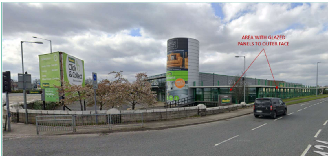
Figure 2.6.4.17 Location of glazed panels at Woodies DIY (Image source: Google)
