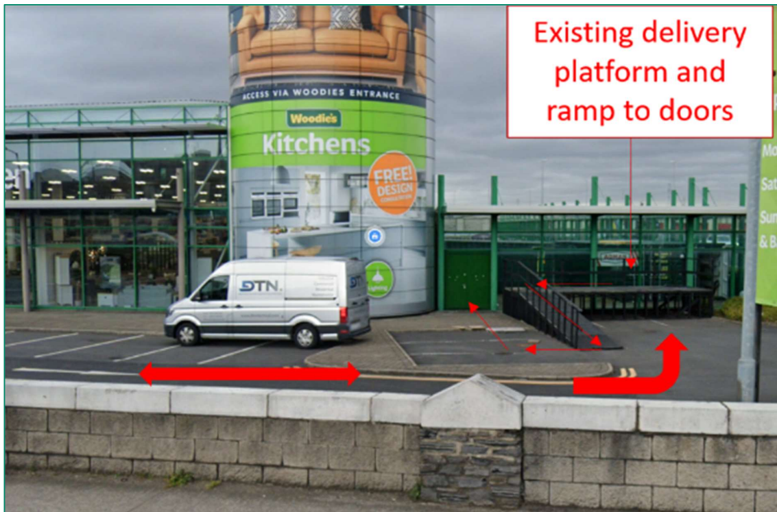
Figure 2.6.4.7: Existing delivery platform and ramp (Image source: Google)
