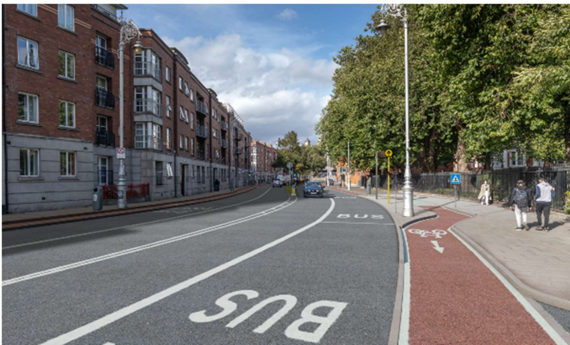
Figure 2.8.12.6: Extract from Photomontage View 18 As Proposed View from South along Patrick Street (Figure 17.2.18.2)
