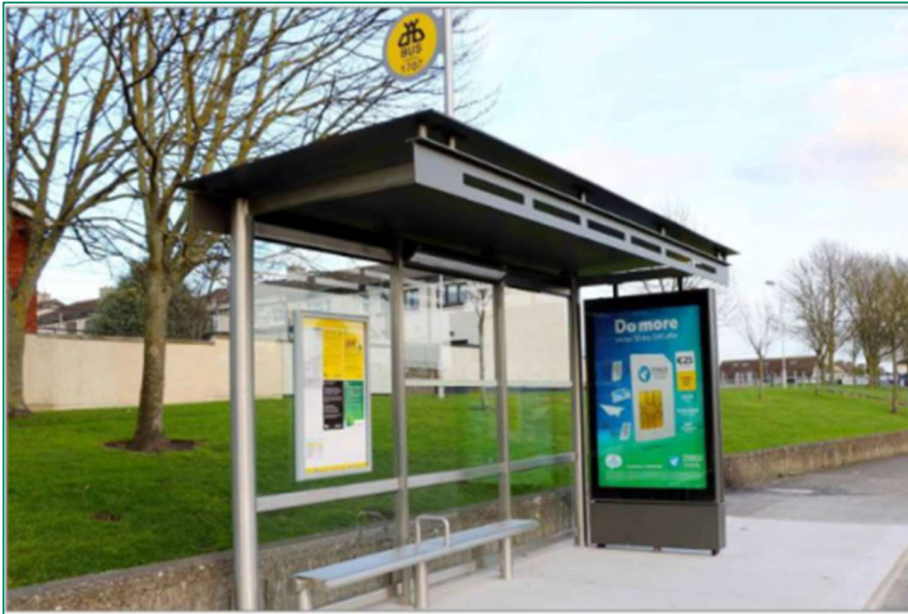
Figure 2.8.12.1: Standard 3 Bay Reliance Mark Shelter with full width advertising panel
