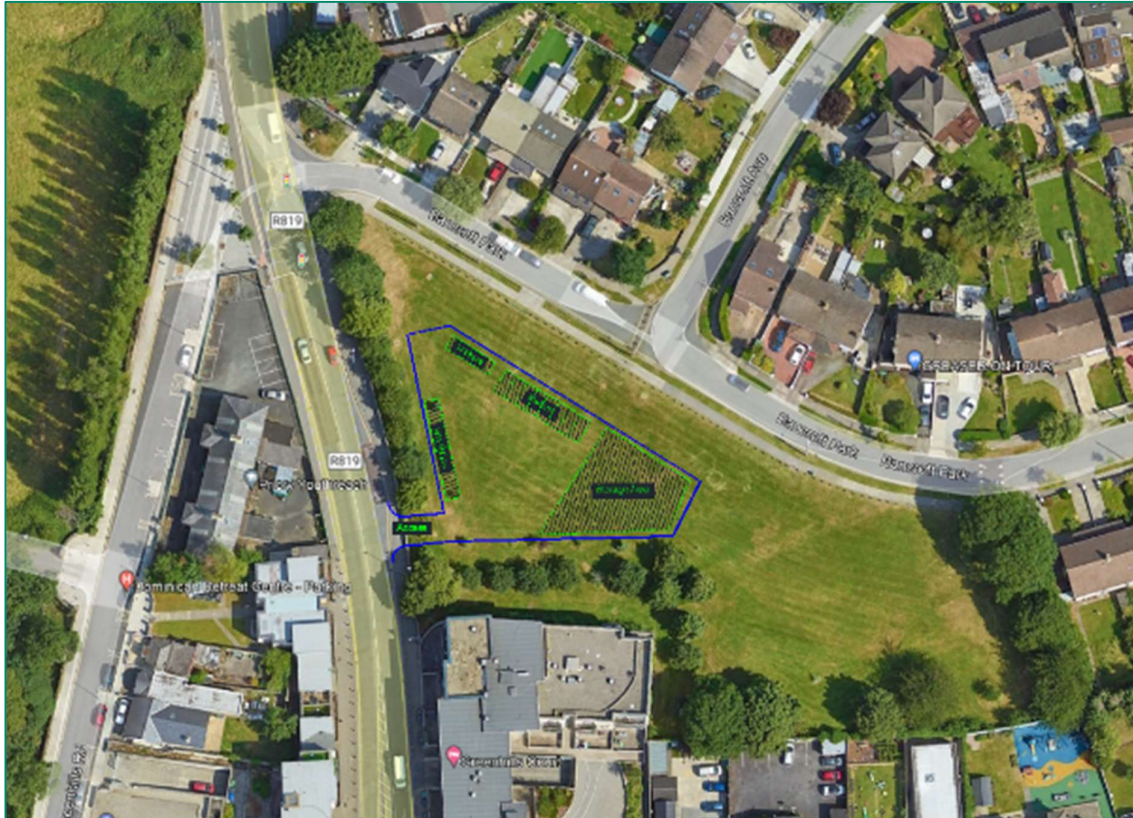
Figure 2.1.6: Site Compound TC2 within the wider green area at Bancroft Park (Image Source: Google)
