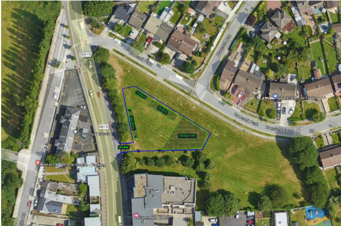
Figure 2.8.11.2: Site Compound TC2 within the wider green area at Bancroft Park (Image Source: Google)
