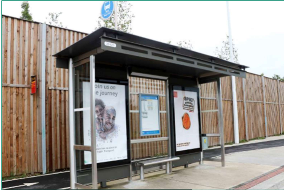
Figure 2.8.12.2: Example of a 3-Bay Reliance Cantilever Shelter with full width roof and half end panels (source: JC Decaux)
